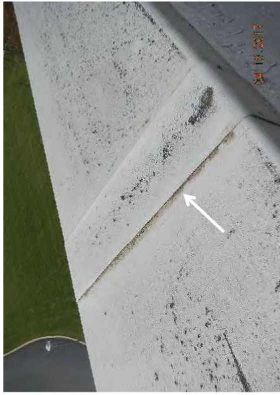
Photo 7 – View of Homogeneous Sampling Area #3, white caulk on metal parapet cap.
