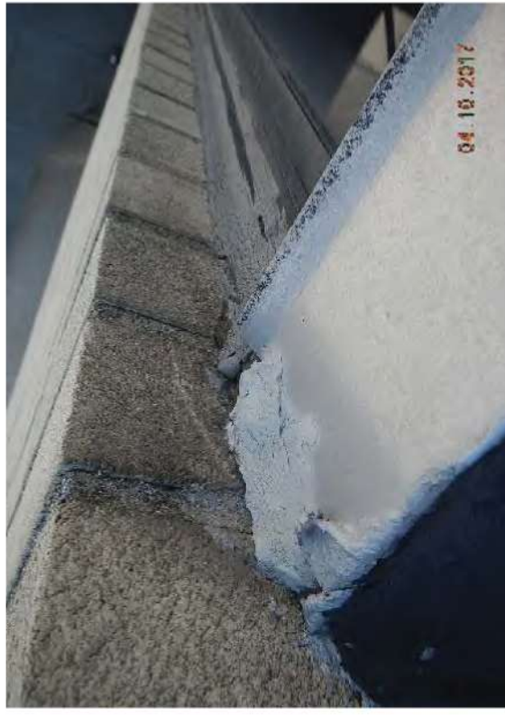
Photo 11 – View of Homogeneous Sampling Area #6, gray and brown parapet wall caulking.
