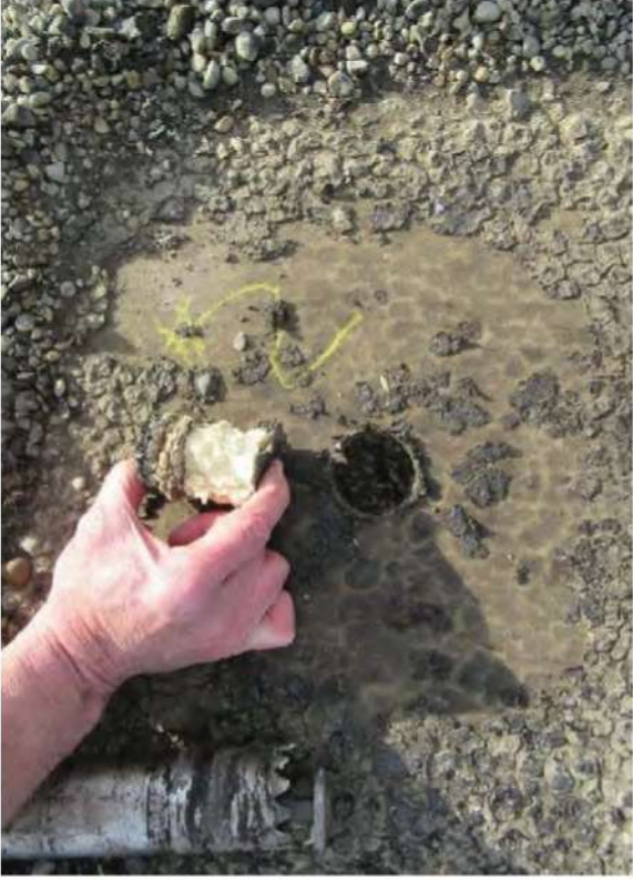
Photo 13 – View of Homogeneous Sampling Area #8, roofing – field.
