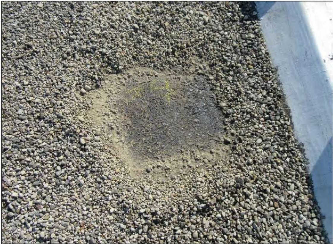
PHOTO #17: Core Cut #9 – View of Core Cut #9 location adjacent parapet wall.
