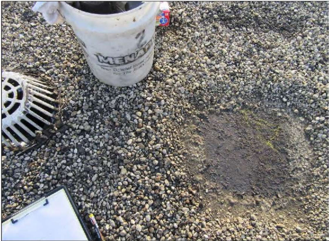
PHOTO #1: Core Cut #1 – View of Core Cut #1 location adjacent roof drain.
