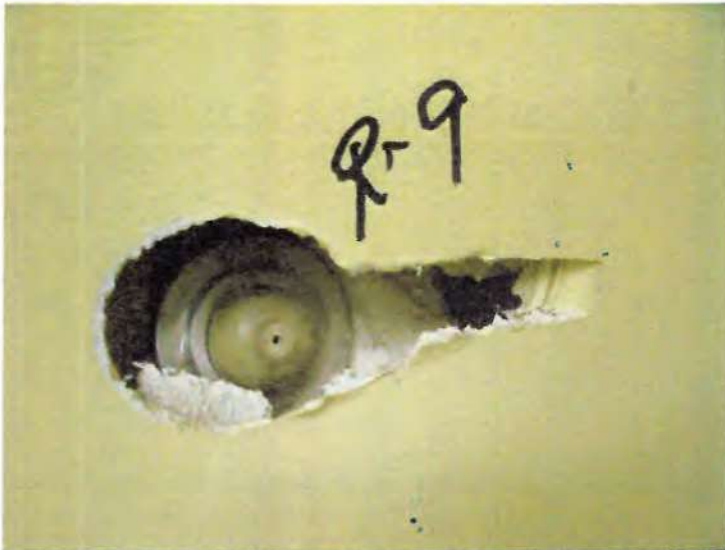
Photo 9: Drywall/JC (R-9) Mail Room. No Asbestos Detected.
