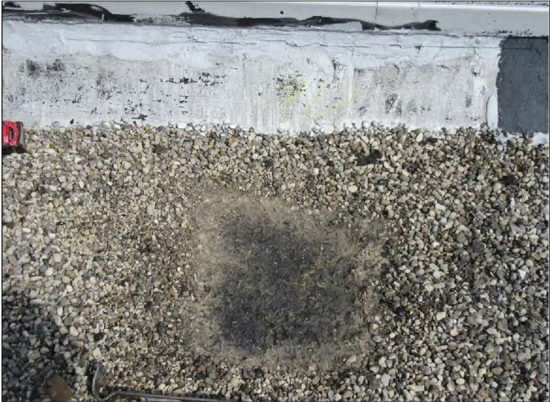
PHOTO #23: Core Cut #12 – View of Core Cut #12 location adjacent parapet wall.
