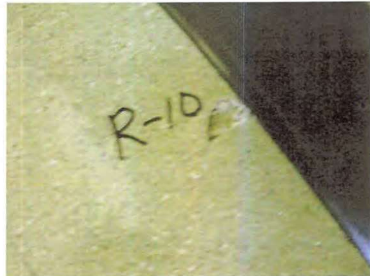
Photo 10: Gray Floor Tile (R-10) Mail Room. No Asbestos Detected.
