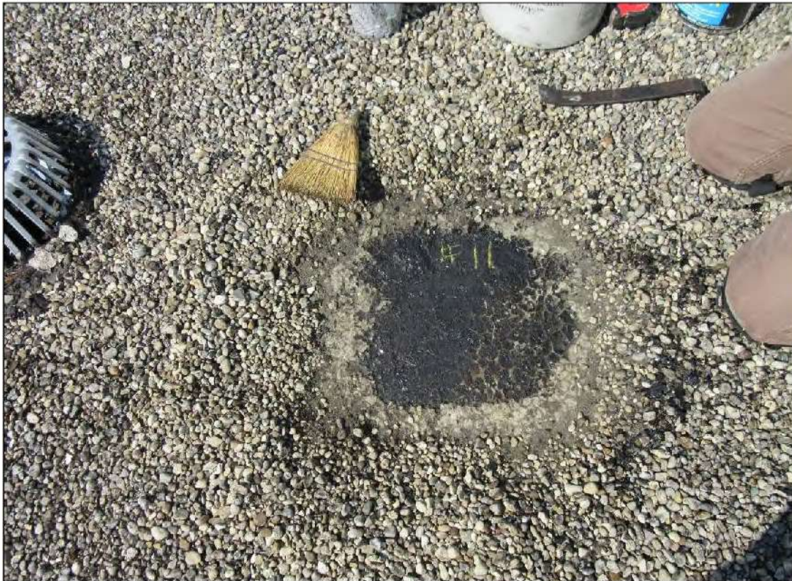
PHOTO #21: Core Cut #11 – View of Core Cut #11 location adjacent roof drain.
