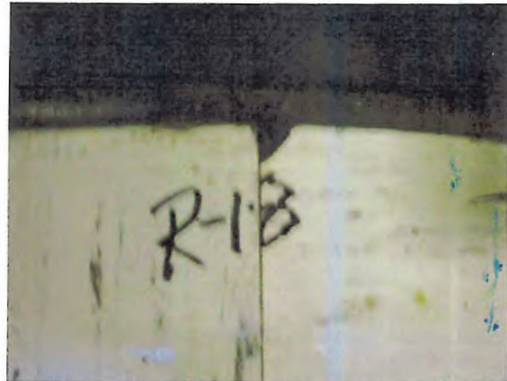
Photo 18: Off-White Floor Tile (R-18) Room 226. 2% Chrysotile Asbestos Detected (.50% Point Count). Off-White Floor Tile Mastic, 7.50% Chrysotile Asbestos Detected.
