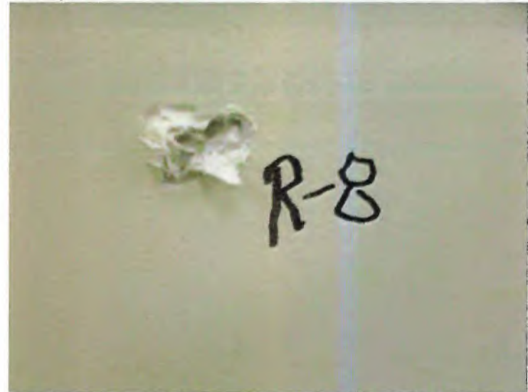
Photo 8: Drywall/JC (R-8) Hallway. No Asbestos Detected.
