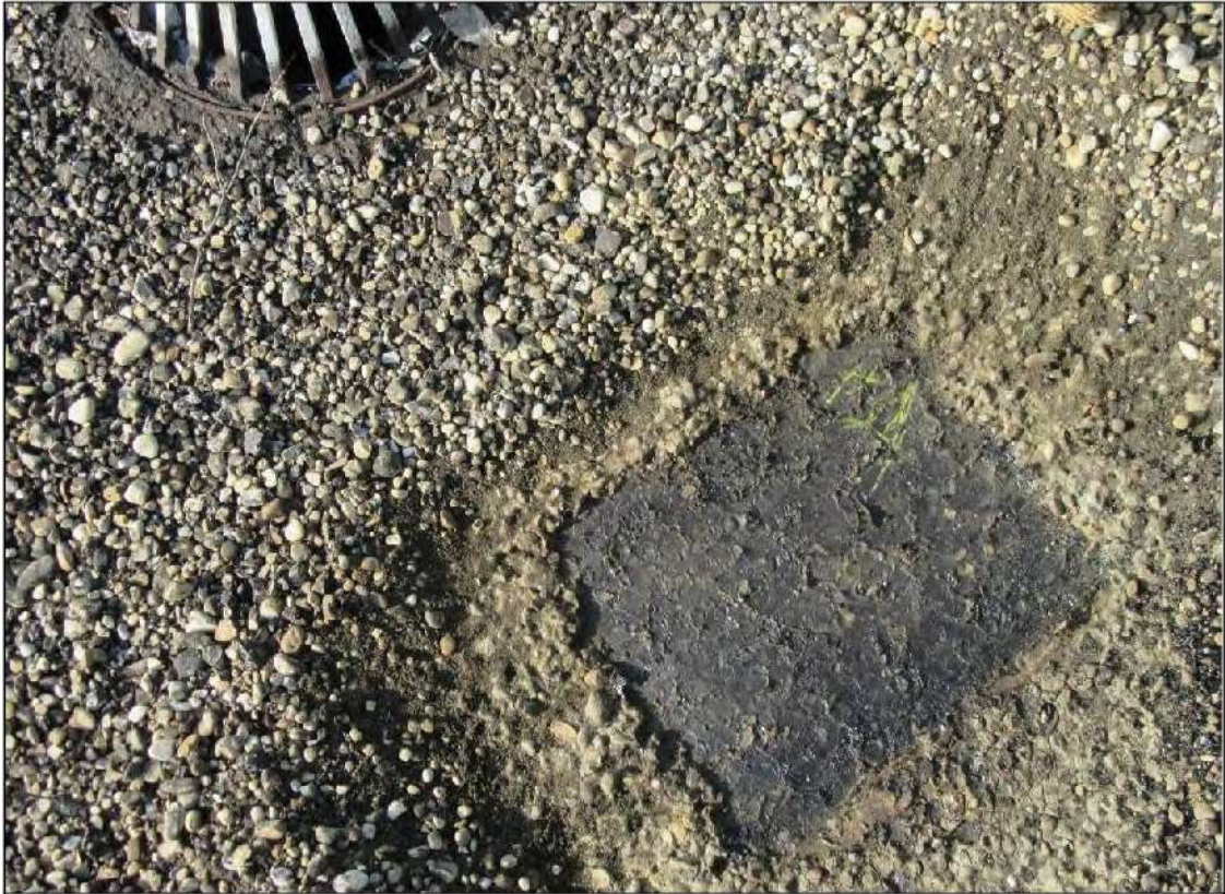
PHOTO #7: Core Cut #4 – View of Core Cut #4 location adjacent roof drain.
