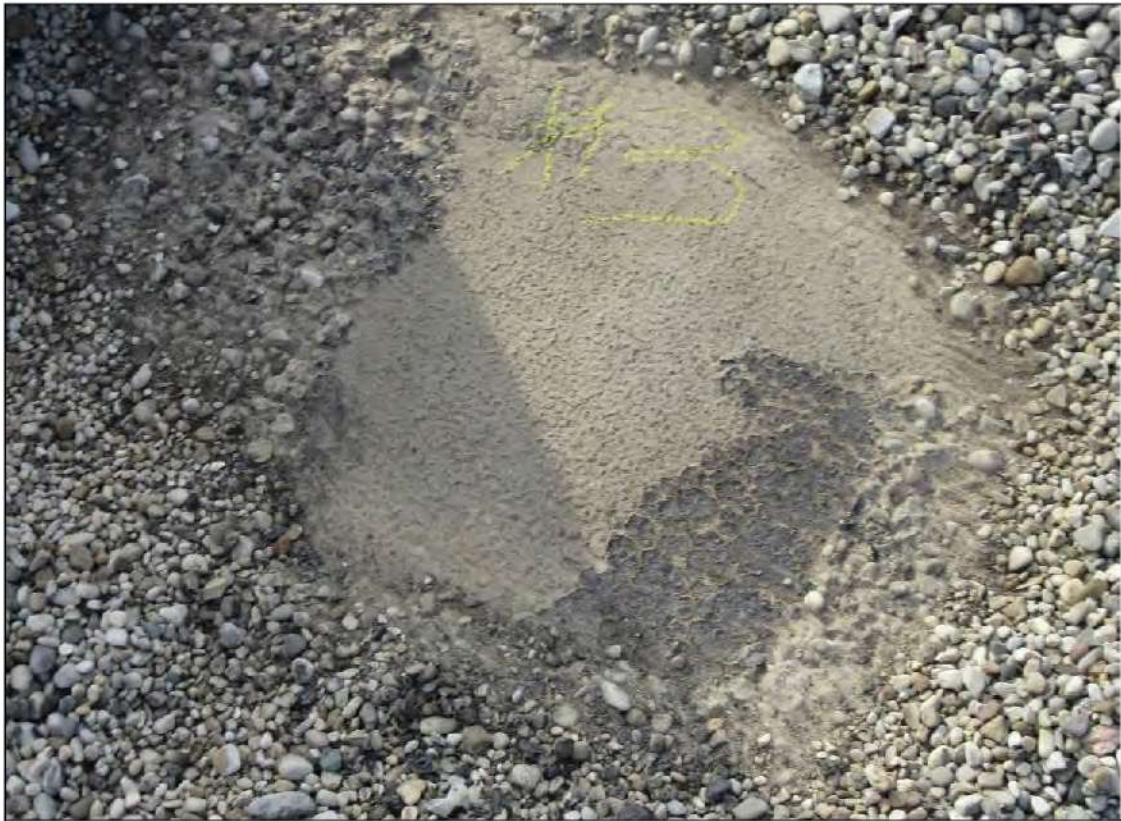
PHOTO #5: Core Cut #3 – View of Core Cut #3 location adjacent parapet wall.
