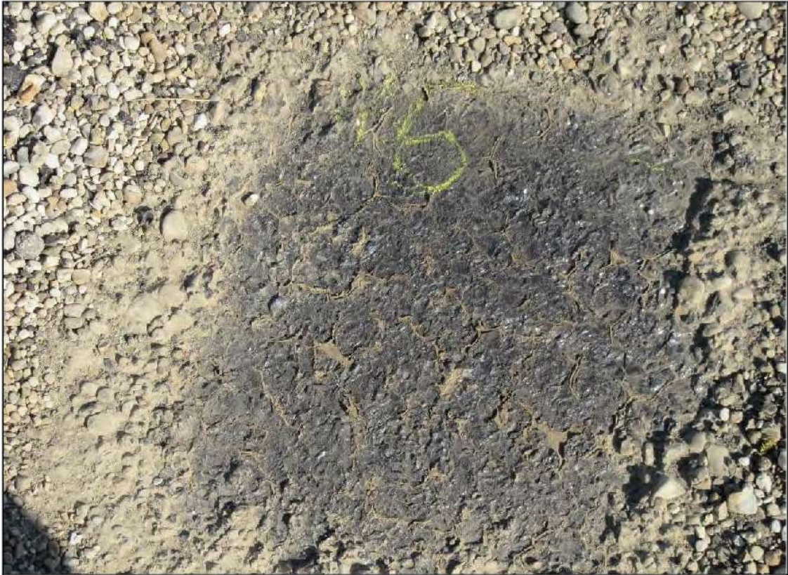
PHOTO #11: Core Cut #6 – View of Core Cut #6 location adjacent parapet wall.
