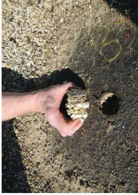
Photo 12 – View of Homogeneous Sampling Area #7, roofing flashing.
