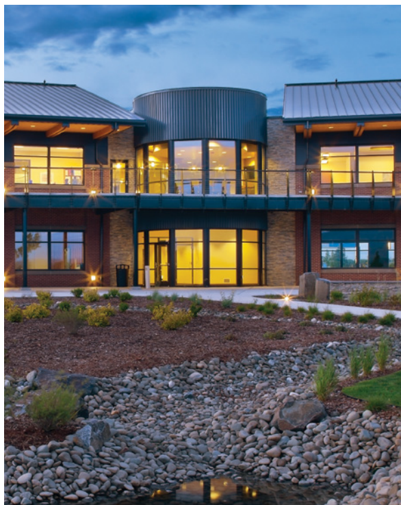
Osprey Pointe, Port of Pasco Headquarters, Pasco, WA Architect: BCRA, Inc.
