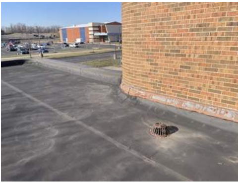
Photo 73- 2nd Floor, Rooftop, All Bituminous Roofing is Assumed to Contain Asbestos
