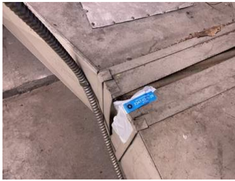
Photo 29- Sample# 7347-03-11-29, No Asbestos Detected in Vibration Isolator Cloth
