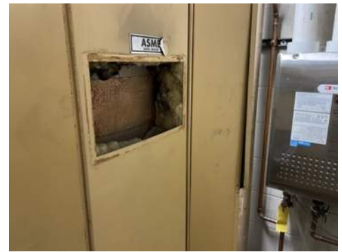
Photo 75- 3rd Floor, Hot Water Heater, Fiberglass Insulation
