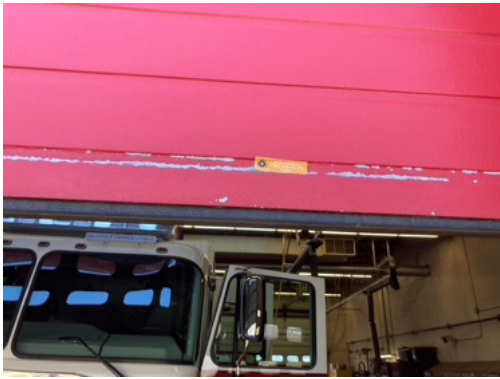
Paint Film Sample 7347-03-11-73 with no detectable lead
