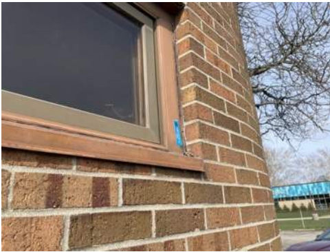
Photo 58- Sample# 7347-04-01-22, No Asbestos Detected in Grey Exterior Caulk
