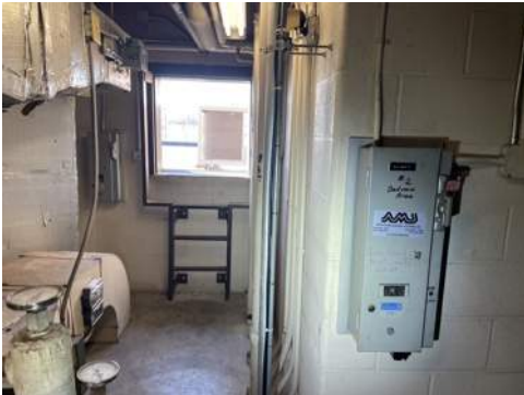
Photo 67- 2nd Floor, Central Tower, SE Area, Safety Switches, All Electrical Insulators are Assumed to Contain Asbestos
