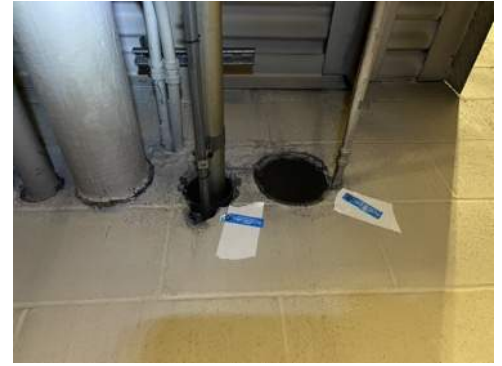
Photo 51- Sample# 7347-04-01-15, 2% Chrysotile Asbestos Detected in Pipe Penetration Caulk
