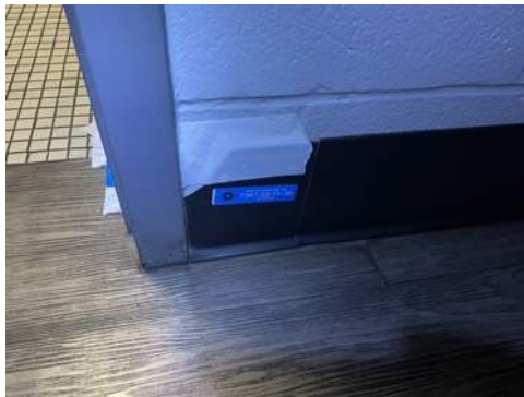
Photo 35- Sample# 7347-03-11-35, No Asbestos Detected in 6" Cove Base and Mastic
