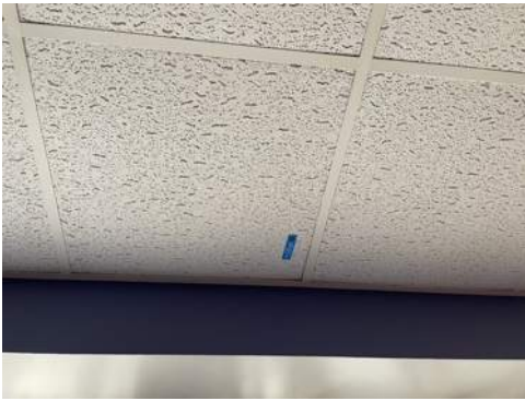
Photo 04- Sample# 7347-03-11-04, No Asbestos Detected in 2' x 2' Ceiling Tile
