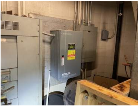
Photo 64- 1st Floor, Central Tower, East Wall, Switch and Circuit Breaker, All Electrical Insulators are Assumed to Contain Asbestos
