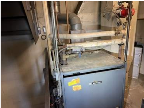
Photo 70- Boiler, Boiler Exhaust Flue is Assumed to Contain Asbestos
