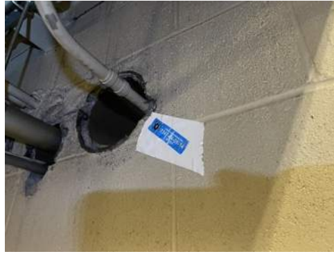
Photo 50- Sample# 7347-04-01-14, 2% Chrysotile Asbestos Detected in Pipe Penetration Caulk
