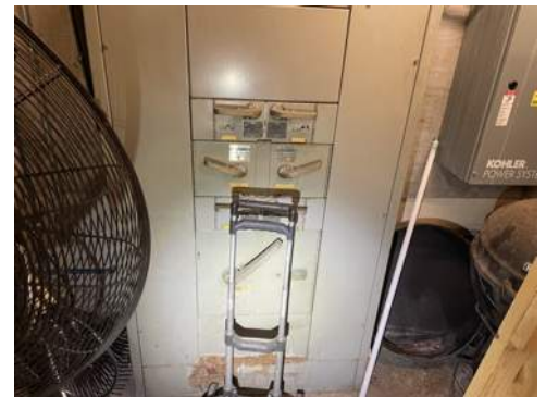
Photo 63- 1st Floor, Central Tower, East Wall, Switch Gear, All Electrical Insulators are Assumed to Contain Asbestos
