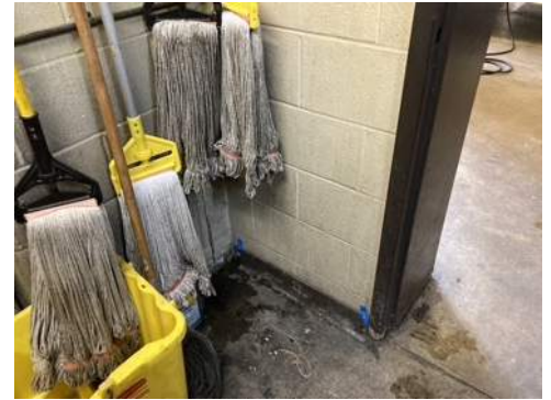
Photo 33- Sample# 7347-03-11-33, No Asbestos Detected in Brown Cove Base Mastic
