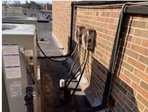
Photo 68- 2nd Floor, Rooftop, S Central Area, Safety Switches, All Electrical Insulators are Assumed to Contain Asbestos
