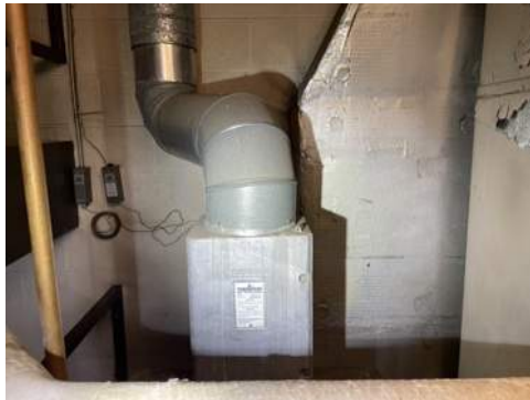
Photo 71- Boiler, Boiler Exhaust Flue is Assumed to Contain Asbestos
