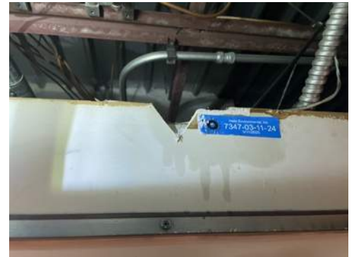
Photo 24- Sample# 7347-03-11-24, No Asbestos Detected in Drywall and Joint Compound
