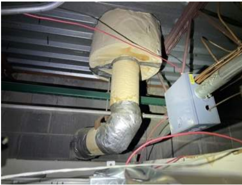
Photo 76- No Visible Hard Pipe Fittings, All Pipe Insulation Sealant is Confirmed to Contain Greater than 1% Asbestos
