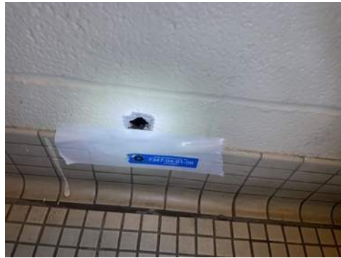
Photo 41- Sample# 7347-04-01-05, No Asbestos Detected in Ceramic Tile, Tan Adhesive, and Grout
