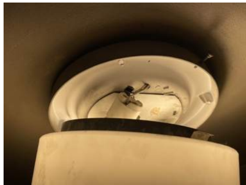
Photo 80- 1st Floor, East Central Janitor's Closet, No Reflector Paper
