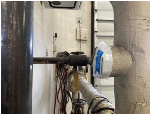
Photo 10- Sample# 7347-03-11-10, 1.1% Chrysotie Asbestos Detected in Grey Pipe Insulation Sealant
