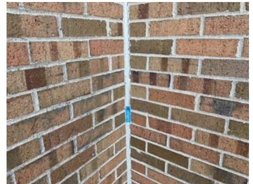
Photo 54- Sample# 7347-04-01-18, No Asbestos Detected in Grey Exterior Caulk
