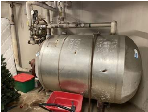
Photo 13- Sample# 7347-03-11-13, 10% Chrysotie Asbestos Detected in Grey Tank Insulation Sealant
