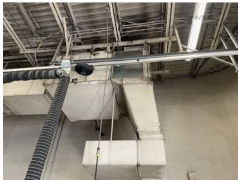
Photo 62- 1st floor, West Vehicle Bay, Southeast Area, All Vibration Isolator Cloths are Assumed to Contain Asbestos, Unless confirmed not to
