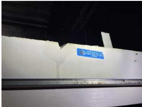
Photo 23- Sample# 7347-03-11-23, No Asbestos Detected in Drywall and Joint Compound
