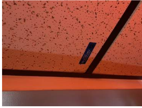
Photo 02- Sample# 7347-03-11-02, No Asbestos Detected in 2' x 2' Ceiling Tile
