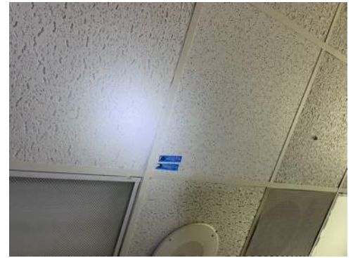
Photo 06- Sample# 7347-03-11-06, No Asbestos Detected in 2' x 2' Ceiling Tile
