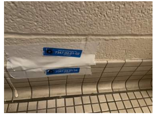
Photo 39- Sample# 7347-04-01-02, No Asbestos Detected in White Concrete Block Coating
