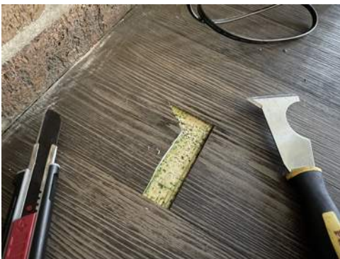
Photo 79- 1st Floor, East Dining Room, Sheet Flooring over <1% Grey 12" x 12" Floor Tile
