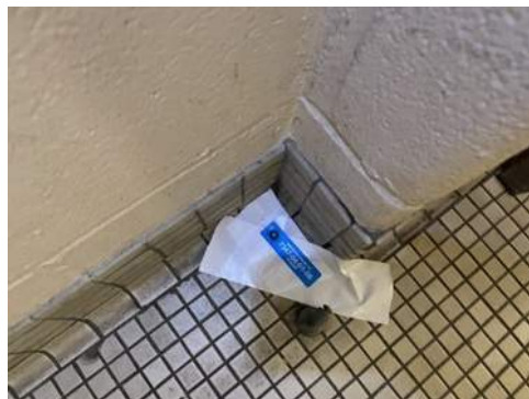
Photo 44- Sample# 7347-04-01-08, No Asbestos Detected in Ceramic Tile, Tan Adhesive, and Grout
