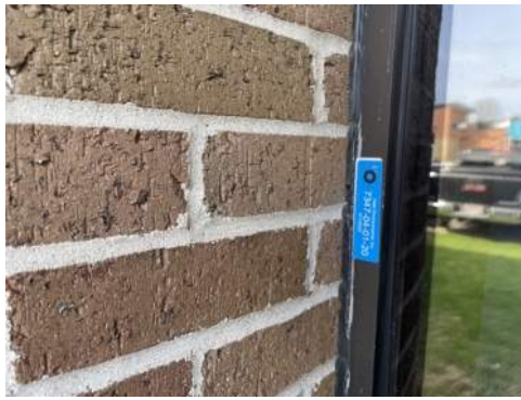
Photo 56- Sample# 7347-04-01-20, No Asbestos Detected in Black Exterior Caulk
