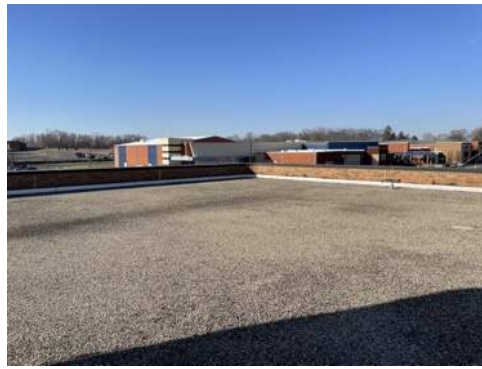
Photo 74- 3rd Floor, Rooftop, All Bituminous Roofing is Assumed to Contain Asbestos
