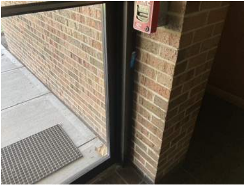
Photo 49- Sample# 7347-04-01-13, No Asbestos Detected in Brown Interior Caulk
