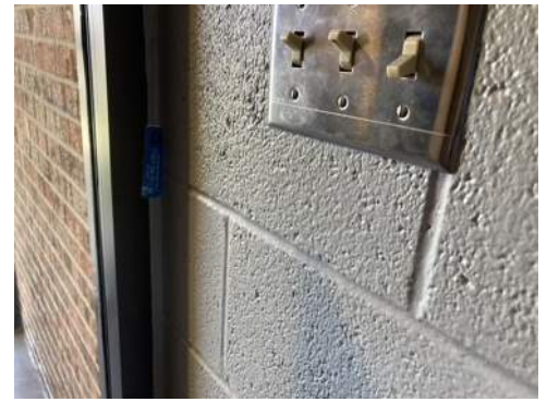
Photo 48- Sample# 7347-04-01-12, No Asbestos Detected in Brown Interior Caulk
