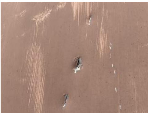
Photo 61- 3rd Floor, Roof Access Door, Visible Insulation, All Insulated Doors are Assumed to Contain Asbestos
