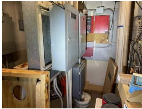
Photo 65- 1st Floor, Central Tower, SE Area, Circuit Breakers, All Electrical Insulators are Assumed to Contain Asbestos
