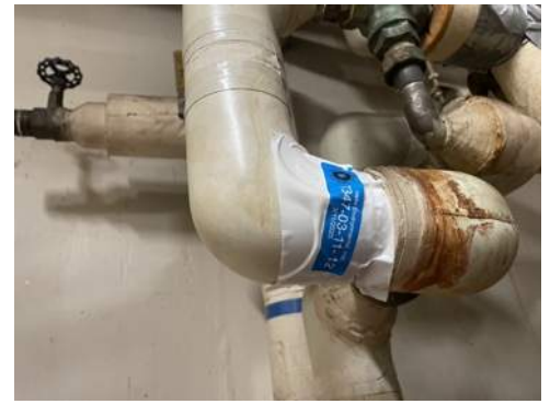
Photo 12- Sample# 7347-03-11-12, 1.6% Chrysotie Asbestos Detected in Tan Pipe Insulation Sealant
