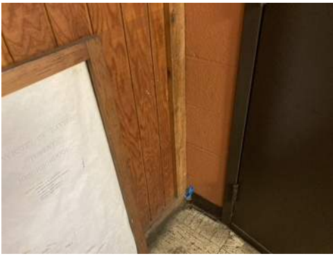
Photo 37- Sample# 7347-03-11-37, No Asbestos Detected in 4" Cove Base and Mastic
