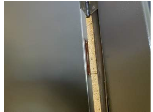
Photo 60- 1st Floor, West Vehicle Bay, Southeast Door, All Fire Doors are Assumed to Contain Asbestos
