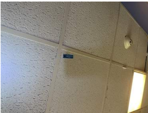
Photo 07- Sample# 7347-03-11-07, No Asbestos Detected in 2' x 2' Ceiling Tile
