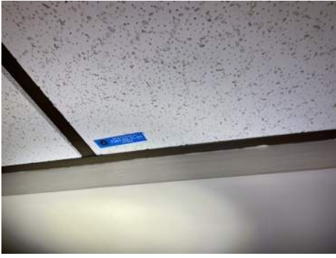
Photo 01- Sample# 7347-03-11-01, No Asbestos Detected in 2' x 2' Ceiling Tile
