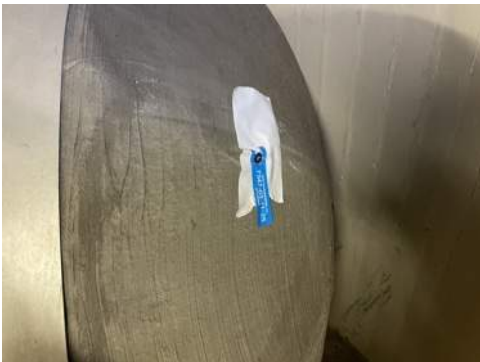
Photo 25- Sample# 7347-03-11-25, 10% Chrysotile Asbestos Detected in Grey Tank Insulation Sealant
