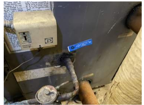
Photo 30- Sample# 7347-03-11-30, No Asbestos Detected in Black Sweat Wrap
