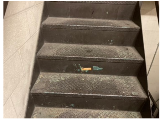
Paint Film Sample 7347-03-11-63 with 0.062% lead
