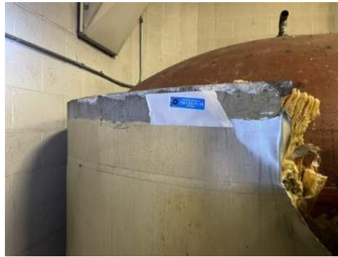
Photo 14- Sample# 7347-03-11-14, 10% Chrysotie Asbestos Detected in Grey Tank Insulation Sealant
