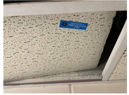
Photo 03- Sample# 7347-03-11-03, No Asbestos Detected in 2' x 2' Ceiling Tile
