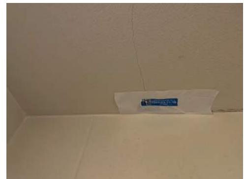
Photo 18- Sample# 7347-03-11-18, No Asbestos Detected in Stucco and Base Layer
