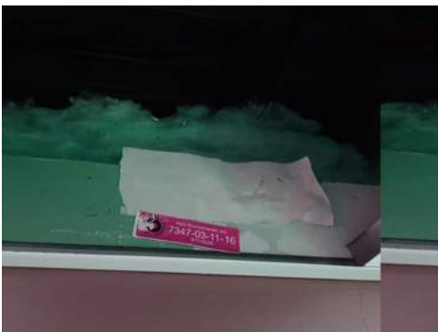
Photo 16- Sample# 7347-03-11-16, No Asbestos Detected in Drywall and Joint Compound
