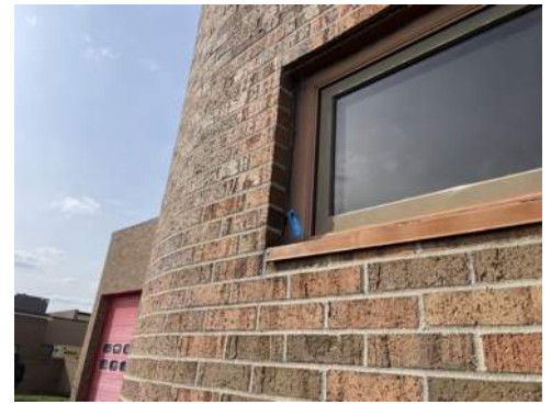
Photo 57- Sample# 7347-04-01-21, No Asbestos Detected in Grey Exterior Caulk
