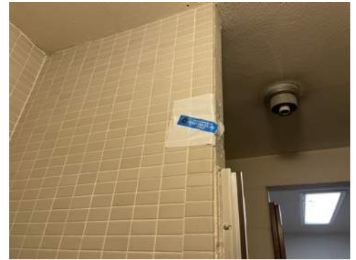
Photo 42- Sample# 7347-04-01-06, No Asbestos Detected in Ceramic Tile, Tan Adhesive, and Grout
