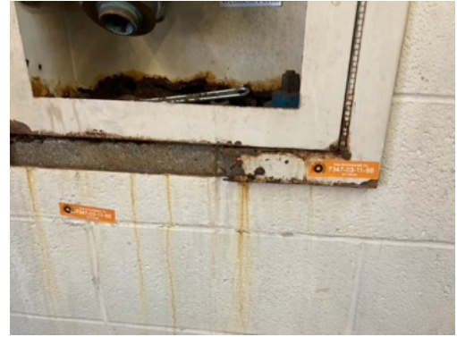
Paint Film Samples 7347-03-11-65 & 66 with no detectable lead
