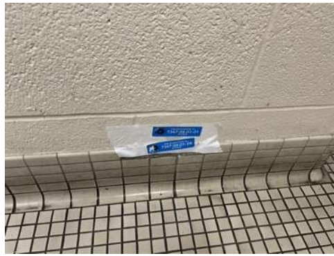
Photo 38- Sample# 7347-04-01-01, No Asbestos Detected in White Concrete Block Coating
