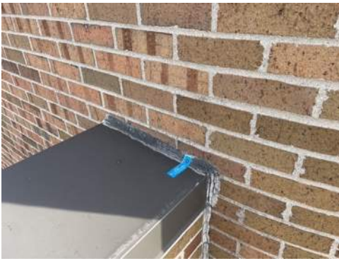
Photo 55- Sample# 7347-04-01-19, No Asbestos Detected in Grey Exterior Caulk
