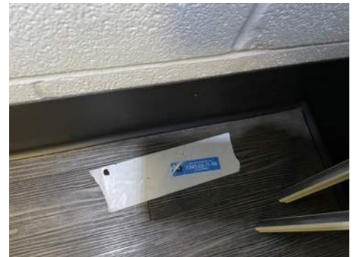
Photo 09- Sample# 7347-03-11-09, No Asbestos Detected in Sheet Flooring and Green Mastic
