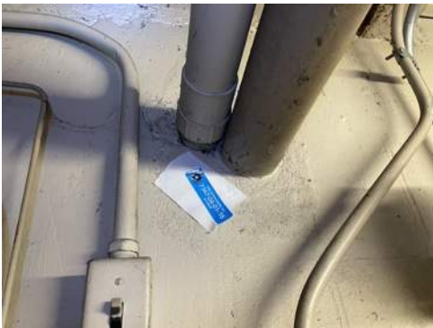
Photo 52- Sample# 7347-04-01-16, No Asbestos Detected in Pipe Penetration Mortar
