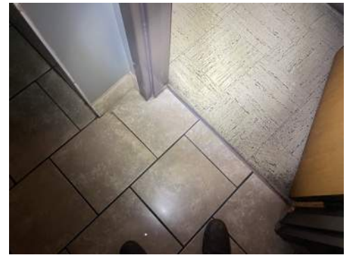
Photo 78- 1st Floor, NE Bathroom, Ceramic Tile over <1% Grey 12" x 12" Floor Tile
