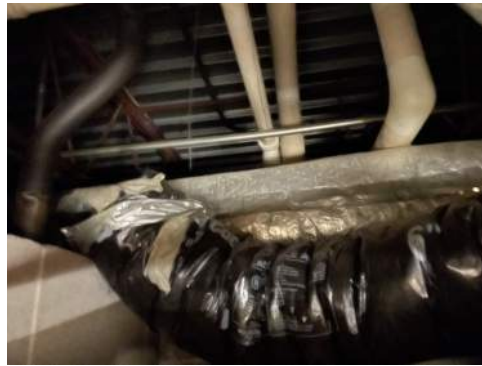
Photo 77- No Visible Hard Pipe Fittings, All Pipe Insulation Sealant is Confirmed to Contain Greater than 1% Asbestos
