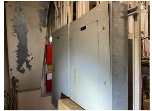
Photo 66- 1st Floor, Central Tower, SE Area, Circuit Breakers, All Electrical Insulators are Assumed to Contain Asbestos
