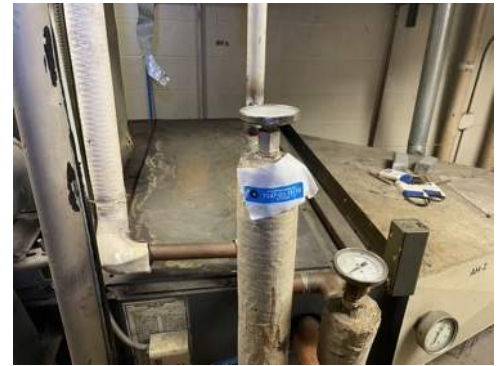
Photo 15- Sample# 7347-03-11-15, No Asbestos Detected in Tan Pipe Insulation Sealant
