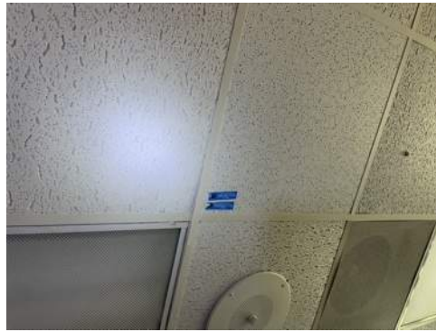
Photo 05- Sample# 7347-03-11-05, No Asbestos Detected in 2' x 2' Ceiling Tile
