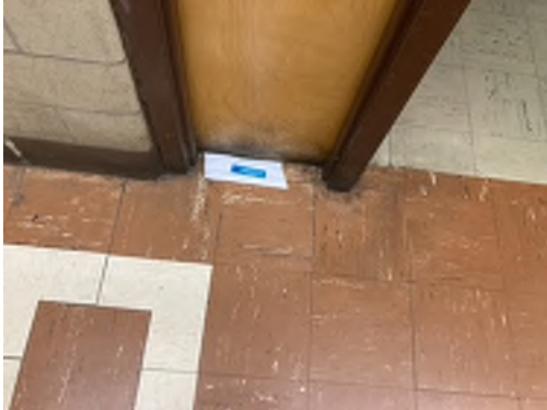
Photo 31- Sample# 7348-03-10-31, 4% Asbestos Detected in 9"x9" Terracotta Streaked Floor Tile, No Asbestos in Black Mastic
