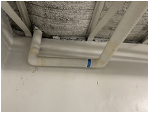
Photo 01- Sample# 7348-03-10-01, No Asbestos Detected in Cream/ Tan Insulation Sealant
