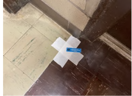
Photo 42- Sample# 7348-03-10-42, 0.5% Asbestos Detected in 9"x9" Maroon Streaked Floor Tile, No Asbestos in Black Mastic
