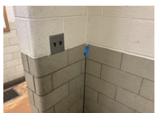
Photo 36- Sample# 7348-03-10-36, 0.9% Chrysotile Asbestos Detected in Grey Interior Caulk
