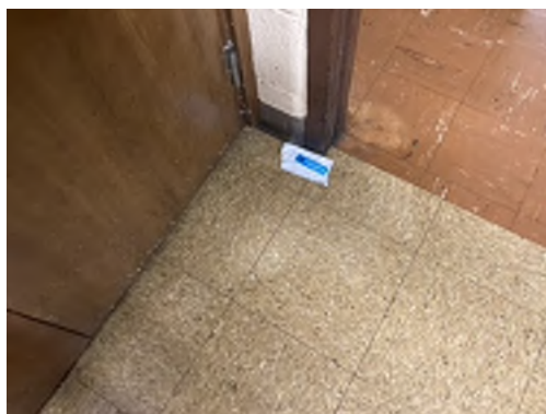
Photo 53- Sample# 7348-03-10-53, No Asbestos Detected in 12"x12" Bronze Mottled Floor Tile and Black Mastic
