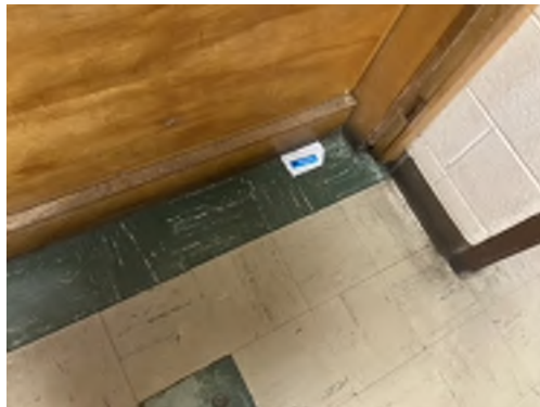
Photo 35- Sample# 7348-03-10-35, 4% Asbestos Detected in 9"x9" Green Streaked Floor Tile, No Asbestos in Black Mastic
