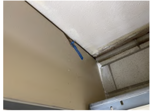
Photo 24- Sample# 7348-03-10-24, No Asbestos Detected in Drywall and Joint Compound
