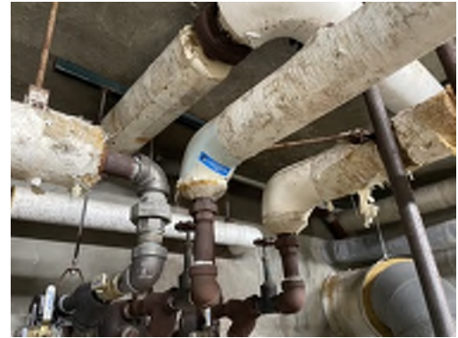
Photo 06- Sample# 7348-03-10-06, No Asbestos Detected in Cream/ Tan Insulation Sealant
