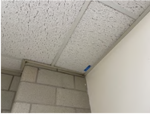
Photo 22- Sample# 7348-03-10-22, No Asbestos Detected in 2' x 2' Ceiling Tile
