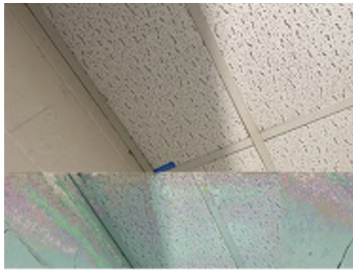
Photo 20- Sample# 7348-03-10-20, No Asbestos Detected in 2' x 4' Ceiling Tile
