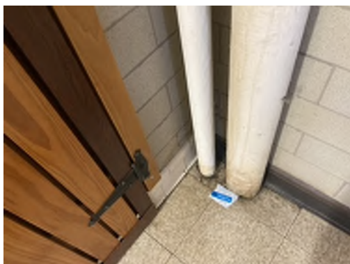
Photo 49- Sample# 7348-03-10-49, No Asbestos Detected in 12"x12" Tan Mottled Floor Tile and Black Mastic
