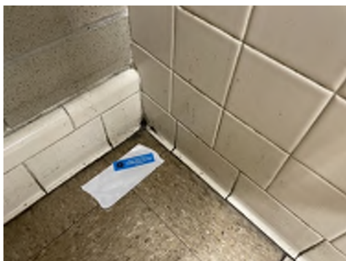
Photo 52- Sample# 7348-03-10-52, No Asbestos Detected in 12"x12" Taupe Mottled Floor Tile and Black Mastic
