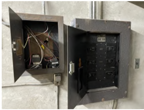
Photo 83- Boiler Room, East Wall, Circuit Breaker, All Electrical Insulators are Assumed to Contain Asbestos
