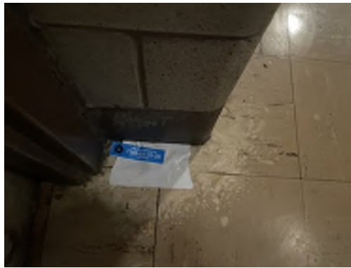
Photo 26- Sample# 7348-03-10-26, 4% Asbestos Detected in 9"x9" Tan Streak Floor Tile, No Asbestos in Black Mastic
