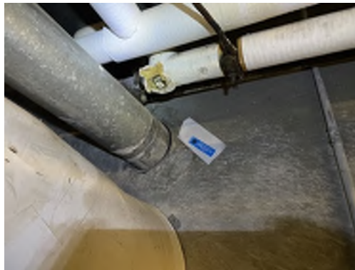
Photo 17- Sample# 7348-03-10-17, No Asbestos Detected in Pipe Penetration Plaster
