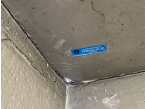
Photo 40- Sample# 7348-03-10-40, No Asbestos Detected in Hard Plaster
