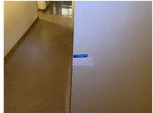
Photo 60- Sample# 7348-03-31-06, No Asbestos Detected in Drywall and Joint Compound
