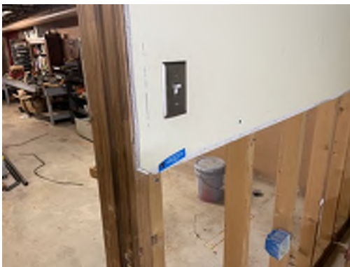
Photo 07- Sample# 7348-03-10-07, No Asbestos Detected in Drywall and Joint Compound
