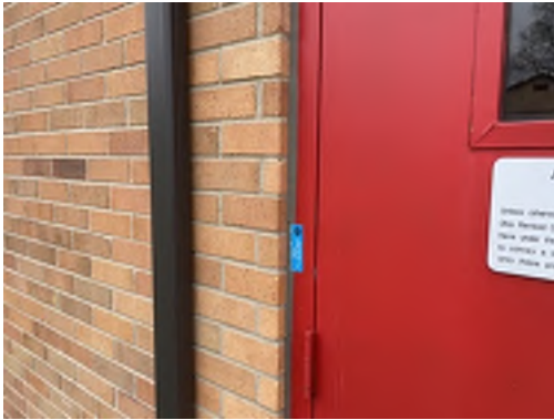
Photo 67- Sample# 7348-03-31-13, No Asbestos Detected in Grey Exterior Caulk
