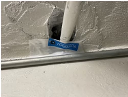
Photo 16- Sample# 7348-03-10-16, No Asbestos Detected in Pipe Penetration Plaster
