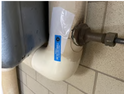
Photo 44- Sample# 7348-03-10-44, No Asbestos Detected in Tan Pipe Insulation Sealant
