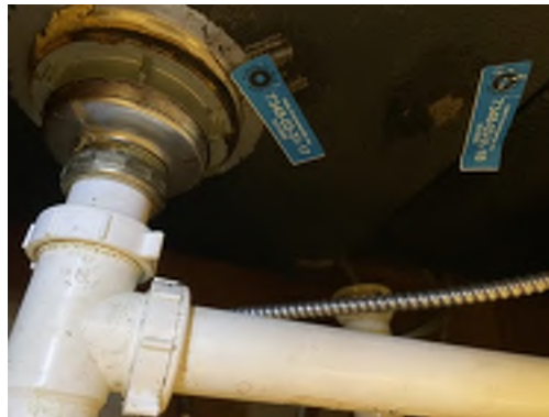
Photo 71- Sample# 7348-03-31-17, No Asbestos Detected in Black Sink Soundproofing
