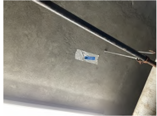
Photo 15- Sample# 7348-03-10-15, No Asbestos Detected in Hard Plaster
