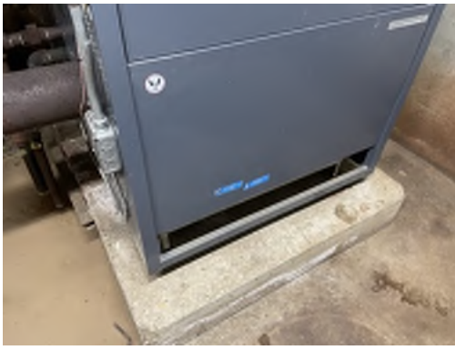
Photo 19- Sample# 7348-03-10-19, No Asbestos Detected in Grey Boiler Sealant
