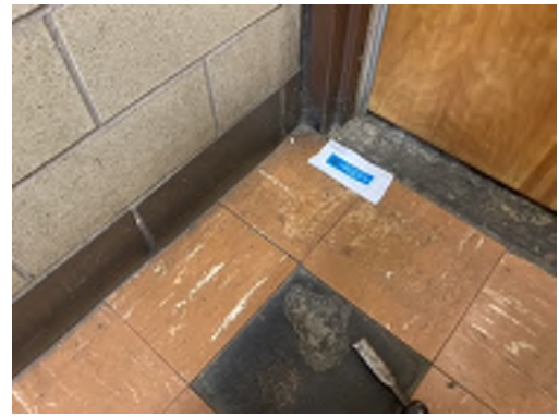
Photo 30- Sample# 7348-03-10-30, 4% Asbestos Detected in 9"x9" Terracotta Streaked Floor Tile, No Asbestos in Black Mastic
