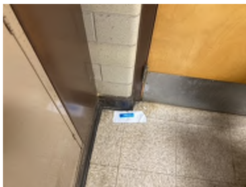
Photo 50- Sample# 7348-03-10-50, No Asbestos Detected in 12"x12" Tan Mottled Floor Tile and Black Mastic
