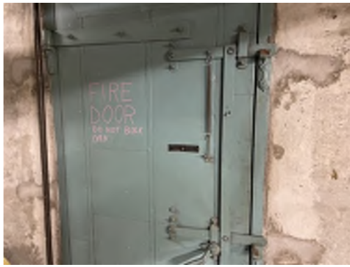
Photo 73- Basement, Boiler Room Entrance Door, All Fire Doors Are Assumed to Contain Asbestos
