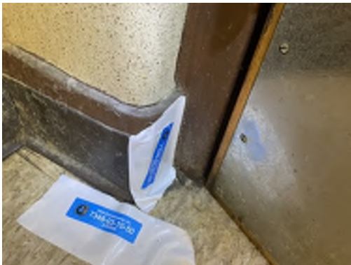
Photo 61- Sample# 7348-03-31-07, No Asbestos Detected in 4" Cove Base and Mastic
