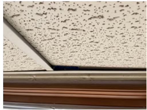
Photo 21- Sample# 7348-03-10-21, No Asbestos Detected in 2' x 4' Ceiling Tile
