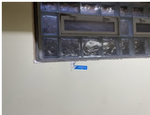
Photo 08- Sample# 7348-03-10-08, No Asbestos Detected in Drywall and Joint Compound
