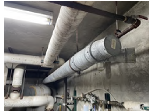
Photo 75- Basement, Boiler Room, Boiler Flue is Assumed to Contain Asbestos, Under the Metal Jacket
