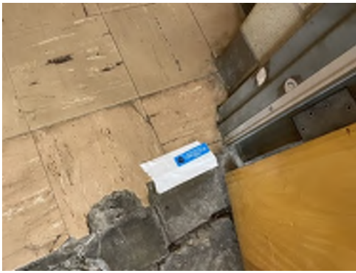
Photo 28- Sample# 7348-03-10-28, 4% Asbestos Detected in 9"x9" Pink Streaked Floor Tile, No Asbestos in Black Mastic
