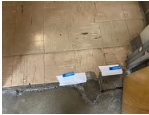
Photo 29- Sample# 7348-03-10-29, 4% Asbestos Detected in 9"x9" Pink Streaked Floor Tile, No Asbestos in Black Mastic
