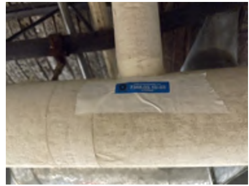
Photo 03- Sample# 7348-03-10-03, No Asbestos Detected in Cream/ Tan Insulation Sealant
