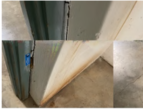
Photo 05- Sample# 7348-03-10-05, 2.5% Chrysotile Asbestos Detected in Grey Interior Caulk
