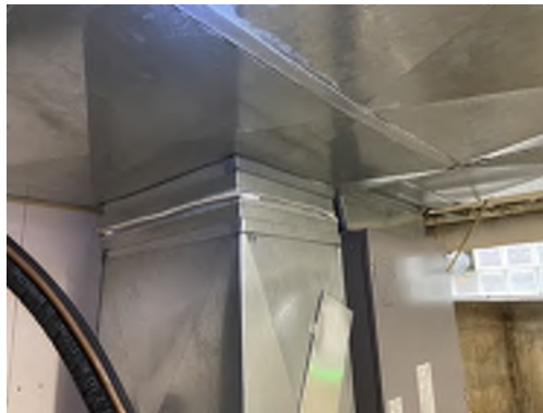
Photo 77- Basement, SW Room, East Area, White Vibration Isolator Cloth is Assumed to Contain Asbestos
