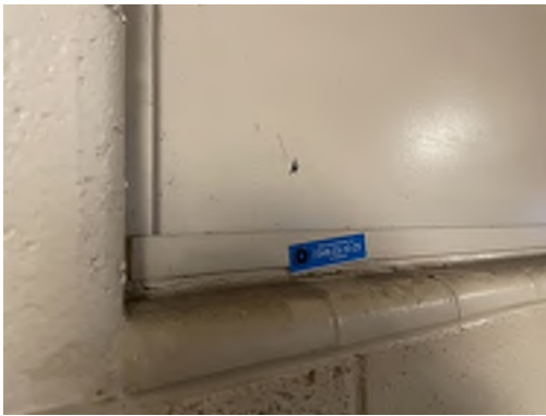
Photo 25- Sample# 7348-03-10-25, 0.3% Chrysotile Asbestos Detected in Grey Interior Caulk
