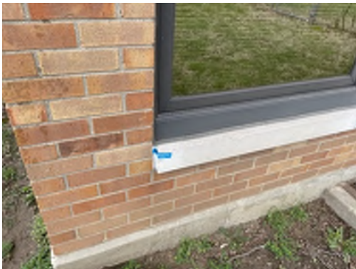
Photo 70- Sample# 7348-03-31-16, No Asbestos Detected in Light Grey Exterior Caulk
