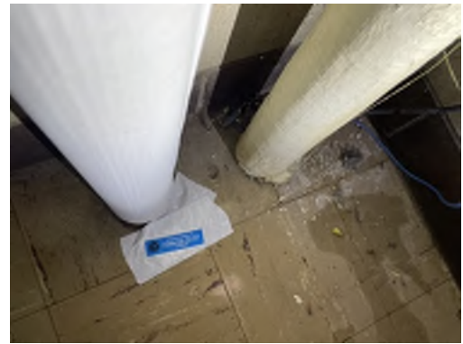
Photo 27- Sample# 7348-03-10-27, 4% Asbestos Detected in 9"x9" Tan Streak Floor Tile, No Asbestos in Black Mastic
