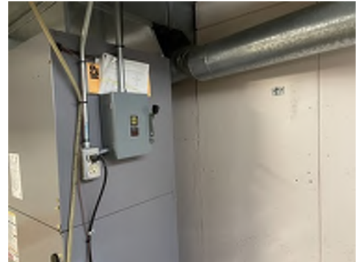
Photo 78- Basement, SW Room, East Area, Electrical Insulators in Safety Switch are Assumed to Contain Asbestos
