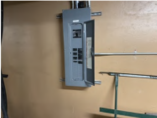
Photo 85- Maintenance Room, South Wall, Circuit Breaker, All Electrical Insulators are Assumed to Contain Asbestos
