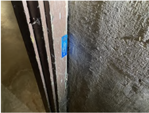
Photo 04- Sample# 7348-03-10-04, 2% Chrysotile Asbestos Detected in Grey Interior Caulk
