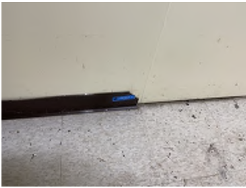
Photo 10- Sample# 7348-03-10-10, No Asbestos Detected in 4" Cove Base and Mastic
