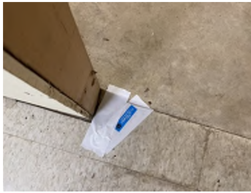
Photo 11- Sample# 7348-03-10-11, No Asbestos Detected in 12" x 12" Tan Mottled Floor Tile and Tan Mastic
