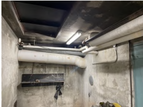
Photo 76- Basement, West Central Hallway, Boiler Flue is Assumed to Contain Asbestos, Under the Metal Jacket
