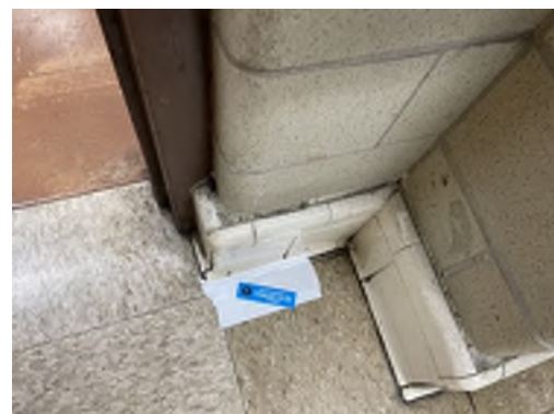
Photo 51- Sample# 7348-03-10-51, No Asbestos Detected in 12"x12" Taupe Mottled Floor Tile and Black Mastic
