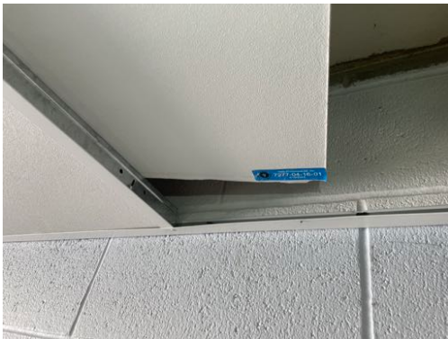
Photo 61- Sample #7277-04-16-01, No Asbestos Detected in Ceiling Tile
