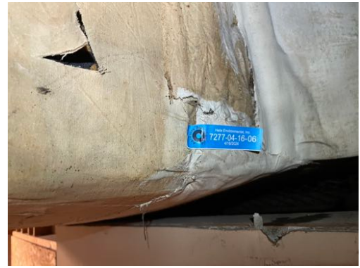
Photo 66- Sample #7277-04-16-06, No Asbestos Detected in White Sealant on Canvas
