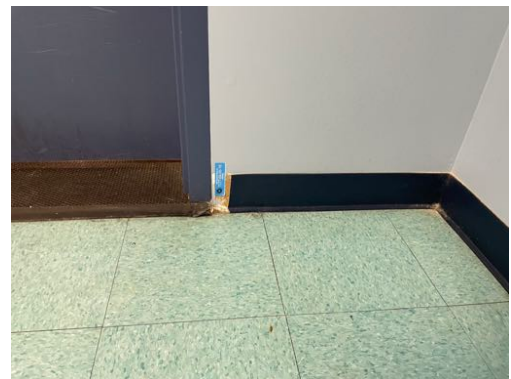
Photo 54- Sample# 7277-04-05-18, No Asbestos Detected in Cove Base and Mastic
