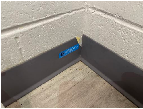
Photo 73- Sample #7277-04-16-13, No Asbestos Detected in Cove Base and Mastic
