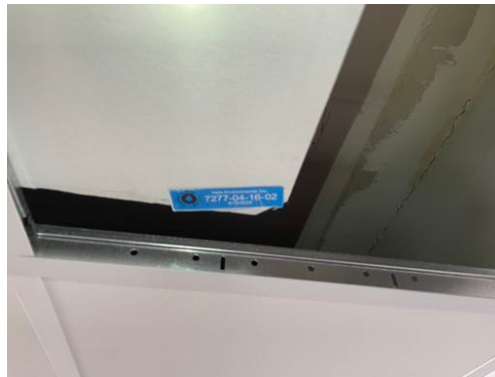
Photo 62- Sample #7277-04-16-02, No Asbestos Detected in Ceiling Tile
