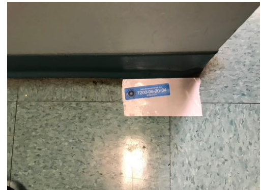
Photo 27- Sample# 7200-06-20-06, No Asbestos Detected in 12"x12" Blue Floor Tile, <1% Asbestos in Black Mastic, Asbestos Floor Tile Beneath
