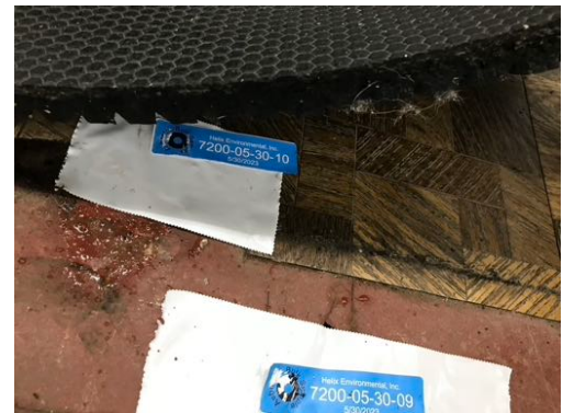
Photo 09- Sample# 7200-05-30-10, No Asbestos Detected in Faux Wood Stick on Floor Tile
