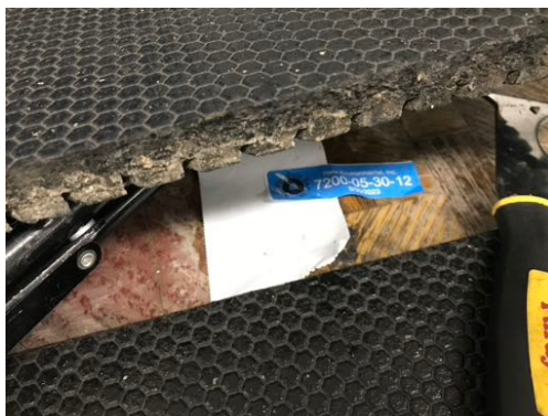
Photo 11- Sample# 7200-05-30-12, No Asbestos Detected in Faux Wood Stick on Floor Tile
