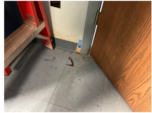
Photo 57- Sample# 7277-04-05-21, No Asbestos Detected in Cove Base and Mastic
