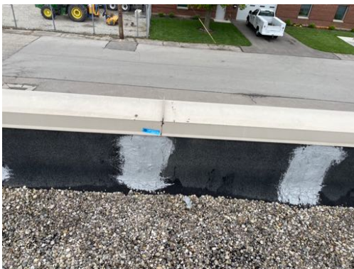
Photo 79- Sample #7277-04-24-02, No Asbestos Detected in Grey Roofing Sealant
