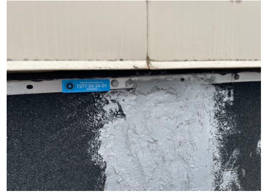
Photo 78- Sample #7277-04-24-01, No Asbestos Detected in Grey Roofing Sealant
