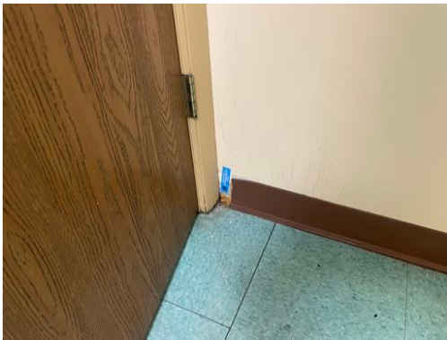
Photo 43- Sample# 7277-04-05-07, No Asbestos Detected in Cove Base and Mastic
