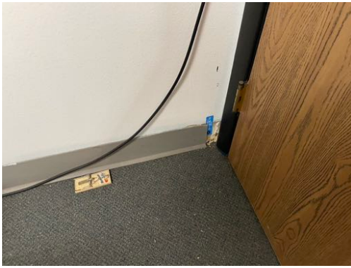
Photo 55- Sample# 7277-04-05-19, No Asbestos Detected in Cove Base and Mastic
