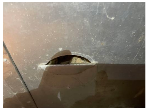
Photo 90- NE Evidence Cooler, Foam Insulation inside of Walk-in Coolers
