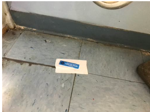
Photo 26- Sample# 7200-06-20-05, No Asbestos Detected in 12"x12" Blue Floor Tile, <1% Asbestos in Black Mastic, Asbestos Floor Tile Beneath
