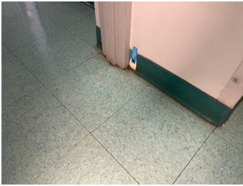
Photo 46- Sample# 7277-04-05-10, No Asbestos Detected in Cove Base and Mastic
