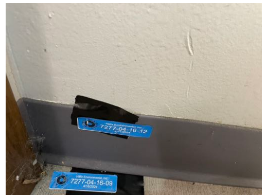
Photo 72- Sample #7277-04-16-12, No Asbestos Detected in Cove Base and Mastic
