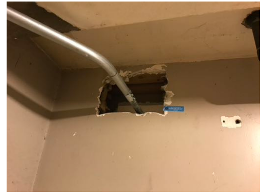
Photo 06- Sample# 7200-05-30-07, No Asbestos in Hard Plaster on Gypsum Lath
