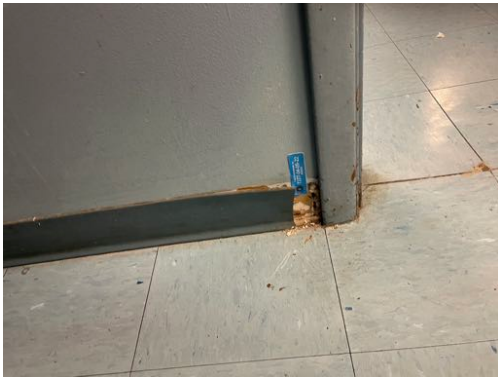
Photo 58- Sample# 7277-04-05-22, No Asbestos Detected in Cove Base and Mastic
