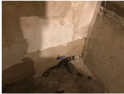
Photo 05- Sample# 7200-05-30-05, No Asbestos in Hard Plaster on Gypsum Lath
