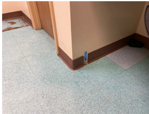
Photo 44- Sample# 7277-04-05-08, No Asbestos Detected in Cove Base and Mastic
