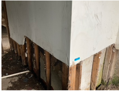
Photo 02- Sample# 7462-03-17-02, No Asbestos Detected in Drywall and Joint Compound
