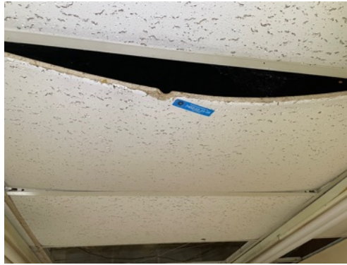
Photo 99 - Sample 7462-03-31-05 with no detectable asbestos
