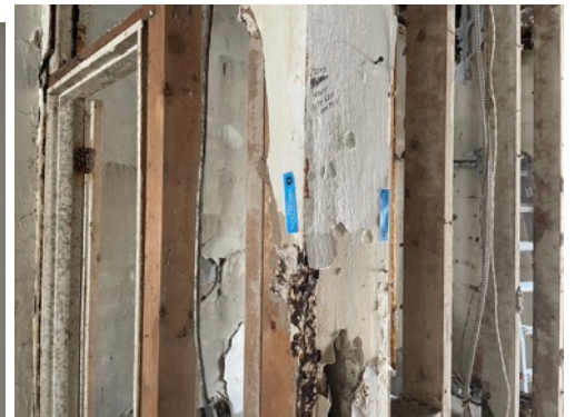
Photo 54 - Samples 7462-03-17-71 and -72 with 3% asbestos in joint compound only
