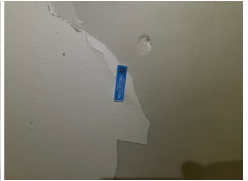
Photo 42 - Sample 7462-03-17-54, No Asbestos Detected
