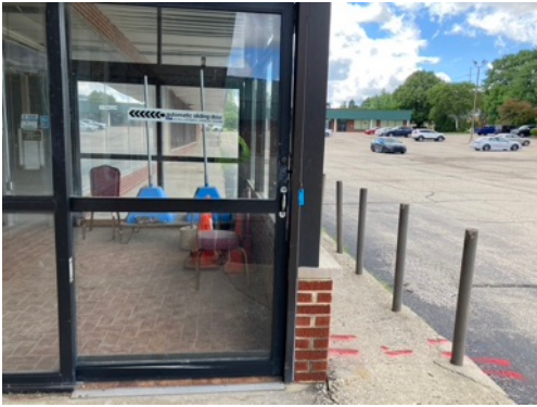
Photo 154 - Sample 7462-04-30-16 with <1% asbestos
