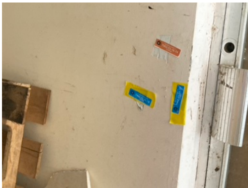
Photo 111 - Samples 7462-03-31-17 and -19 with no detectable asbestos
