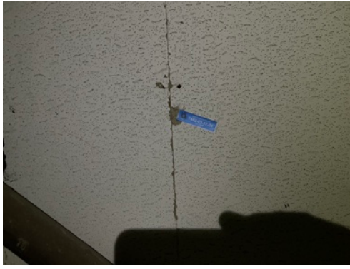
Photo 29 - Sample 7462-03-17-34, No Asbestos Detected
