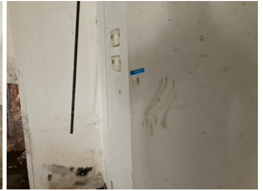
Photo 03- Sample 7462-03-17-03, No Asbestos Detected in Drywall and Joint Compound
