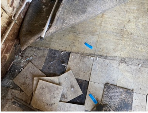
Photo 37 - Samples 7462-03-17-27 and -46 with no detectable asbestos
