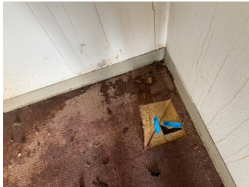
Photo 44 - Samples 7462-03-17-56 and -57 with no detectable asbestos
