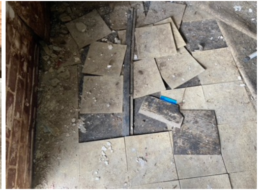
Photo 24 - Sample 7462-03-17-27, 4% Asbestos Detected in tile only
