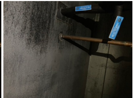
Photo 06- Sample# 7462-03-17-06, No Asbestos Detected in Black Sweat Wrap
