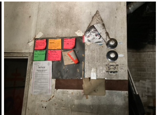
Photo 130 - Mercury-containing thermostats
