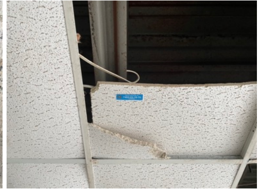
Photo 57 - Sample 7462-03-18-05, No Asbestos
