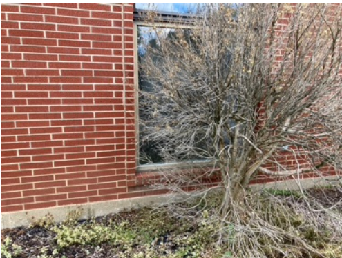
Photo 157 - A Restaurant Windows with Gaskets - No Caulk or Glazing
